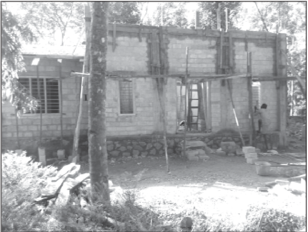
MAKKULAM CHURCH (under construction)
