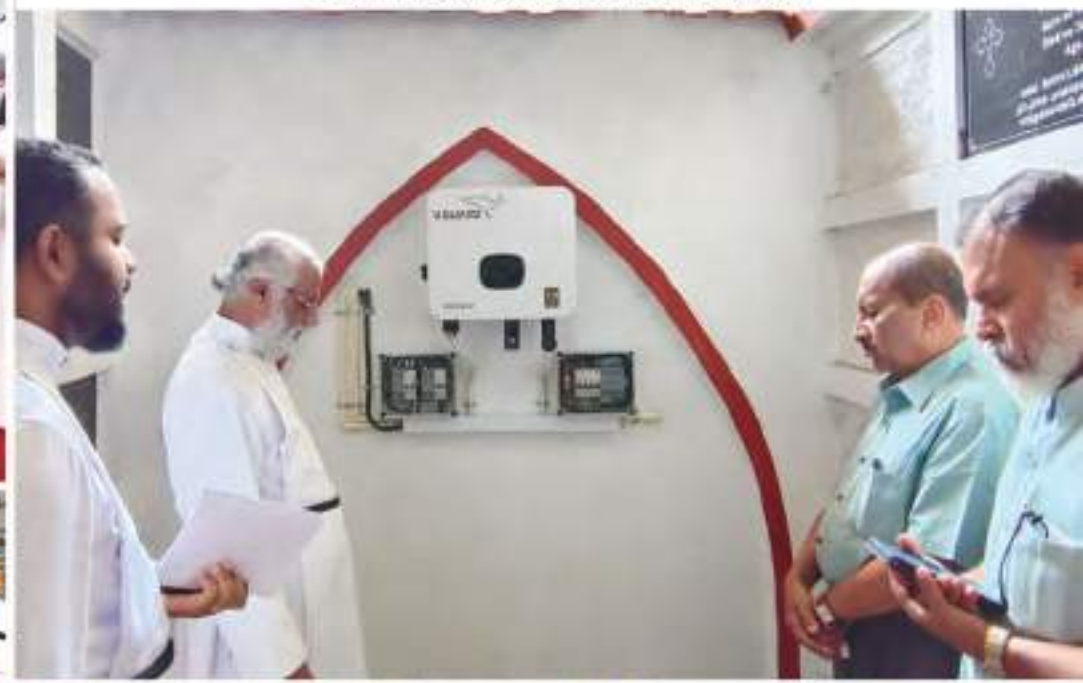
Commissioning of 8KW Solar System
